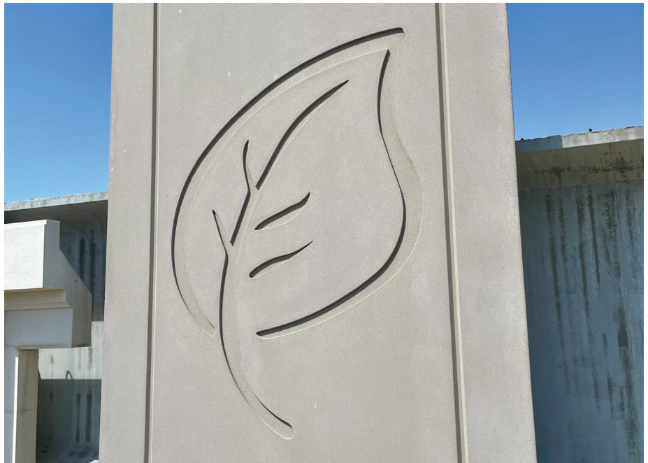
Decorative concrete panel using ASTM C595 Type IP portland-pozzolan cement
